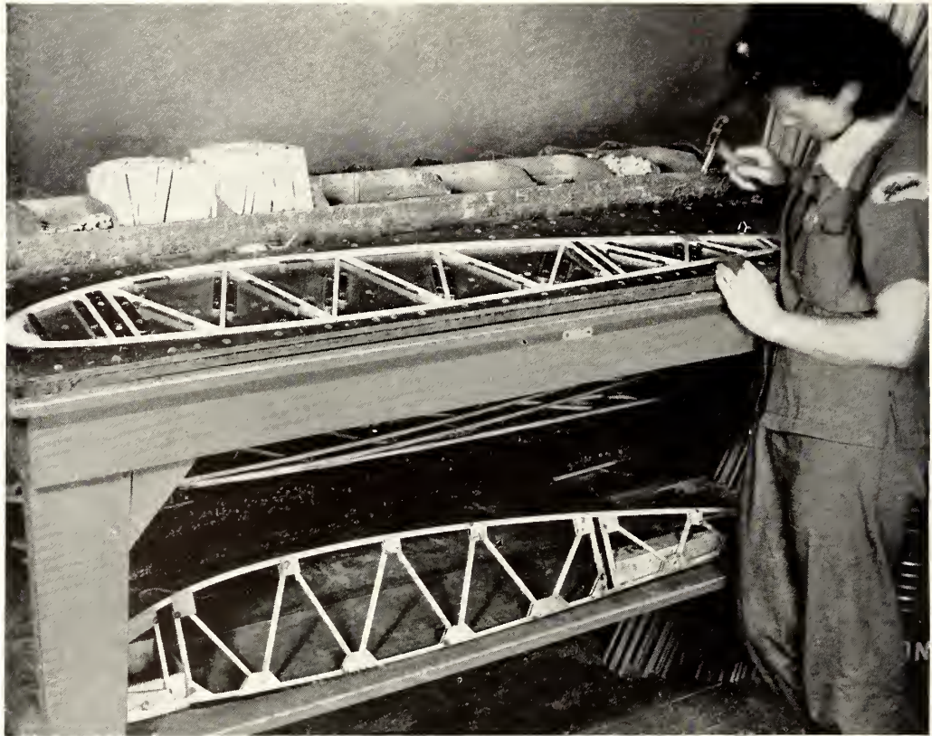
FIGURE 5-42.—Constructing wing ribs by nail gluing.
